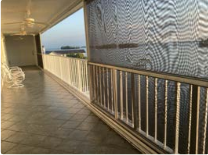
Balcony railings overview
