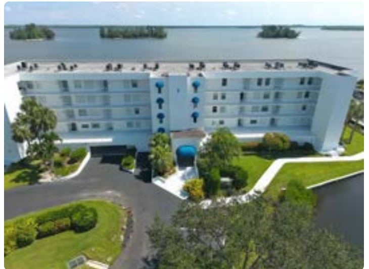
Exterior wall overview
