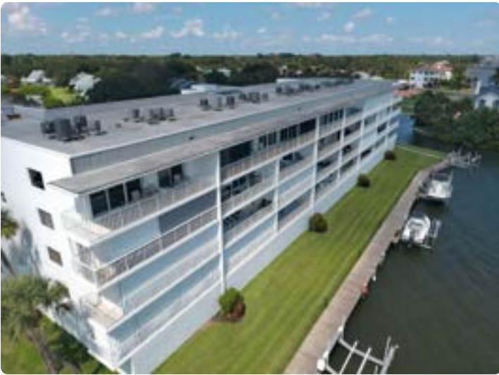
Exterior wall overview
