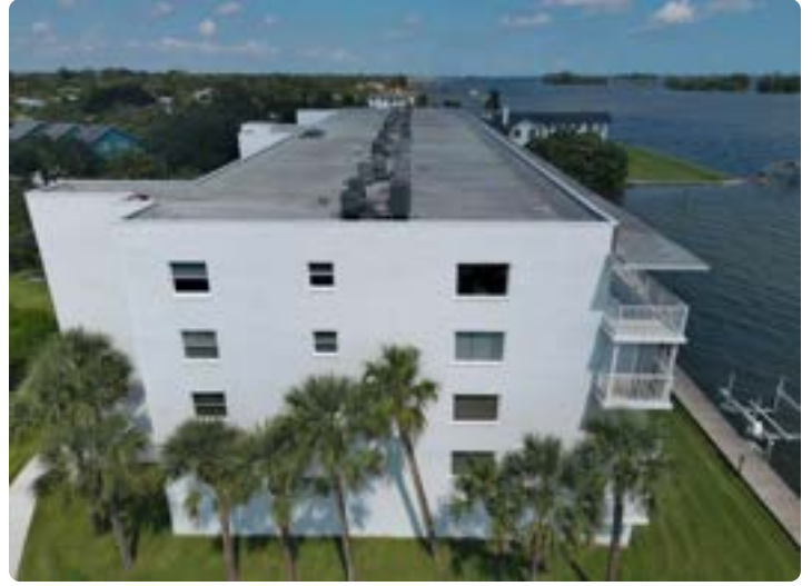
Exterior wall overview
