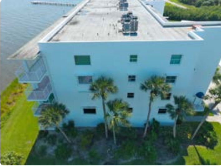
Exterior wall overview
